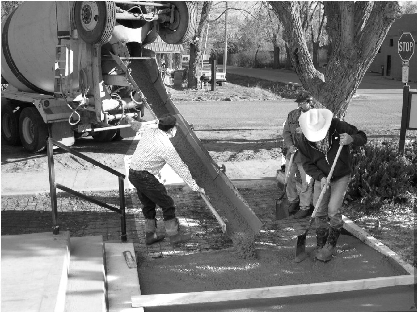
POURING NEW CHURCH STEPS - MARCH 2004
